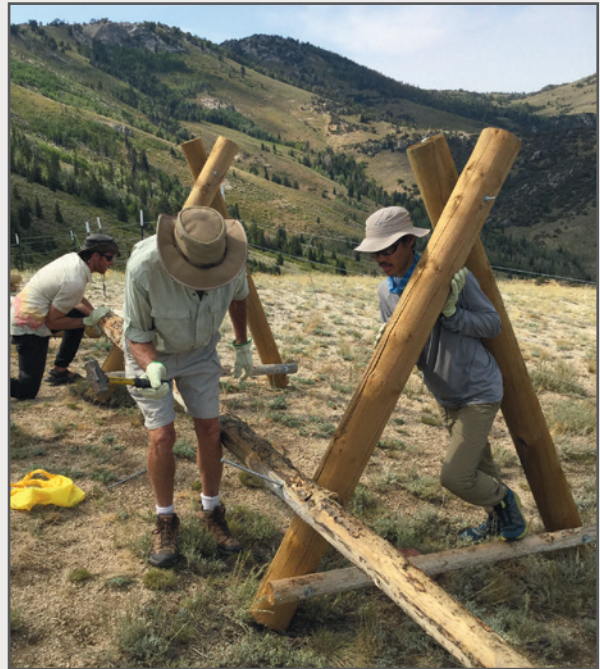
A RECENT CREW CONSTRUCTS BUCK AND RAIL FENCING IN THE DEEP CREEK MOUNTAINS TO PREVENT ILLEGAL TRAVEL INTO THE SCOTT'S BASIN WILDERNESS STUDY AREA. © JEREMY LYNCH/SUWA
