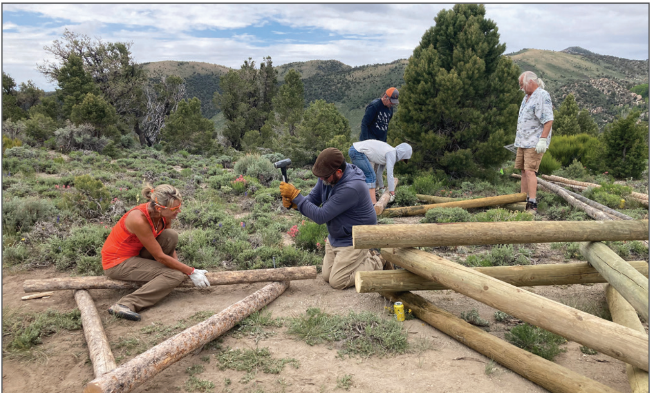
STEWARDSHIP VOLUNTEERS BUILD AND INSTALL BUCK-AND-RAIL FENCING ALONG THE NOTCH PEAK WILDERNESS STUDY AREA BOUNDARY.
