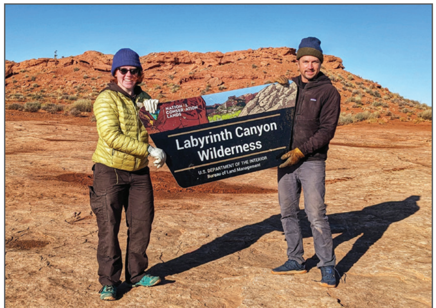
PORTAL SIGNS, AS THEY ARE CALLED, MARK THE BOUNDARIES OF WILDERNESS AREAS AND OTHER PROTECTED LANDSCAPES. THEY ARE USED THROUGHOUT UTAH BY THE BLM. OUR STEWARDSHIP CREWS HAVE HELPED INSTALL SEVERAL OVER THE YEARS. © SUWA
